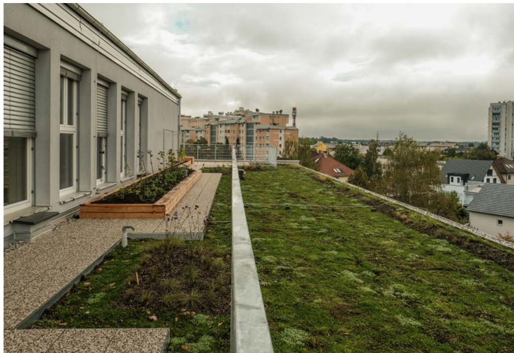
Green roof on Stane Žagar Primary School (photo Jana Jocif)
